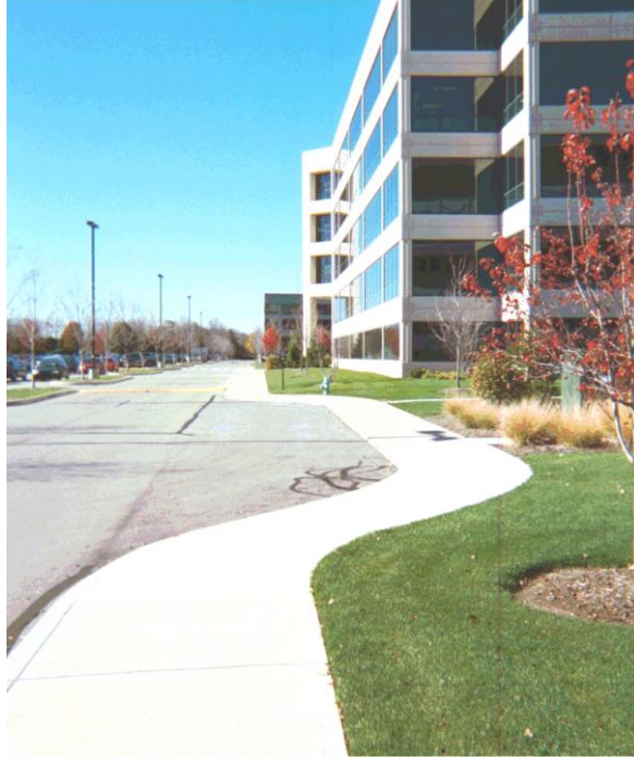
Pull-Off Loading Area
