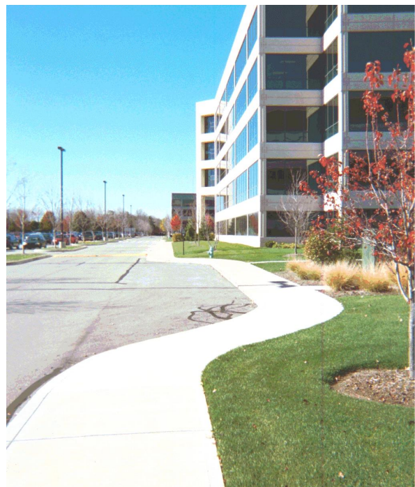
Pull-Off Loading Area
